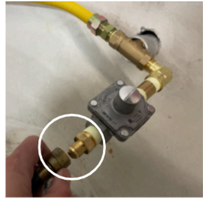
Gas Supply Line to the RV47 Regulator Note: Installer to supply gas line
