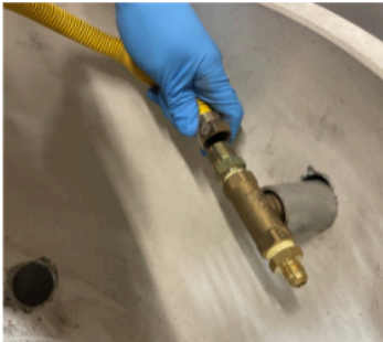
Yellow Flex Line (One End) to Ball Valve
