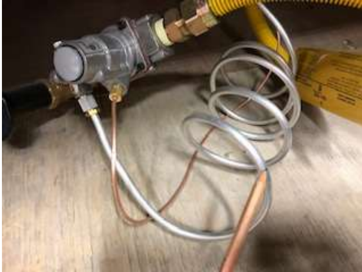
Inlet Tube pictured below the Universal Pilot
